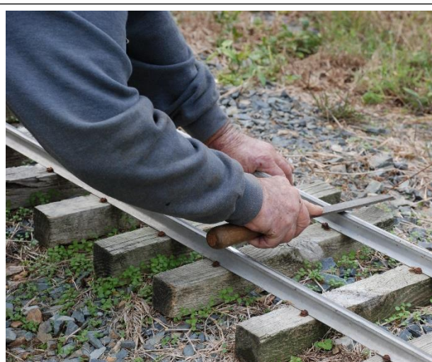
A large file guided by a practiced hand corrects the rail burr caused by the derailment.
