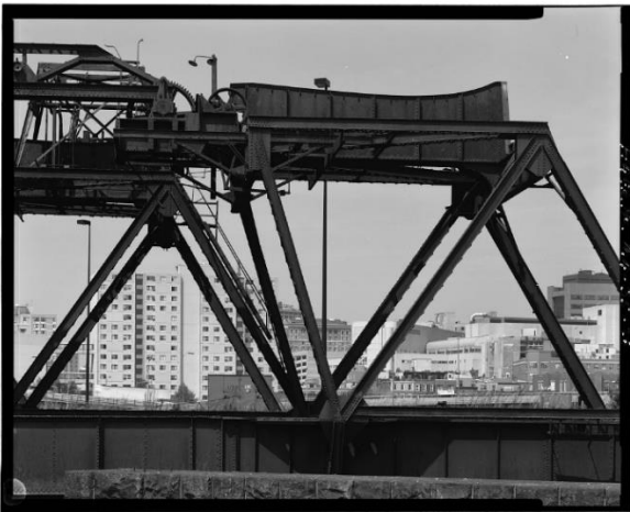
Photo 16: Photo of the operating structure and machinery.
