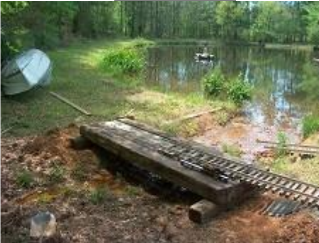
Setting railroad ties for Spillway Bridge.
