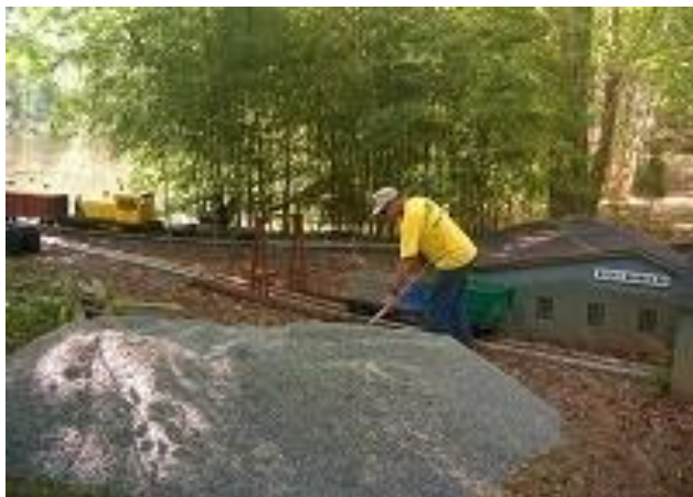
Tons of gravel were used to ballast the track.
