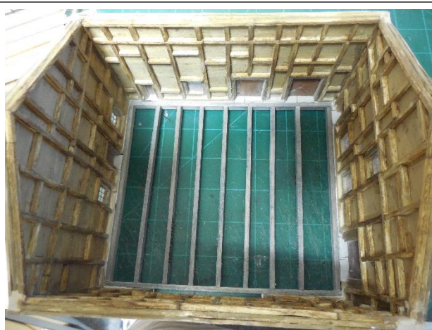
Pic 16: Floor framing with perimeter and joists in place.
