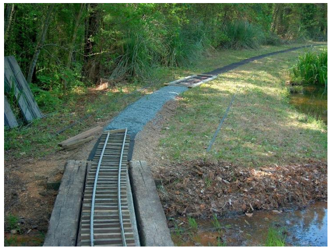
Continuing ballast on down the line.
