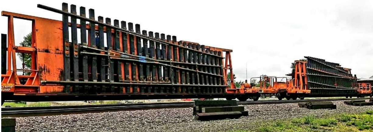
Prefabricated turnouts loaded onto specialized flat cars and ready for installation.
