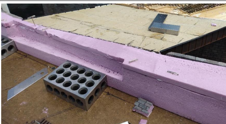
Pic 1: A 1/4" piece of foam was added to bring the height of the abutment filler piece to match the retaining wall height. T-pins hold it in position while the adhesive dries.
