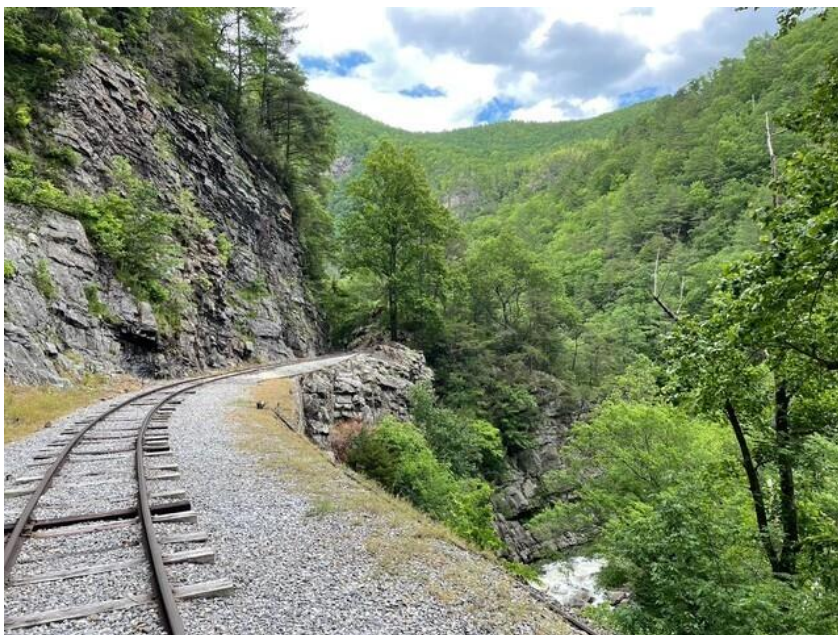
ET&WNC trackage crossed rugged terrain through the Doe River Gorge
