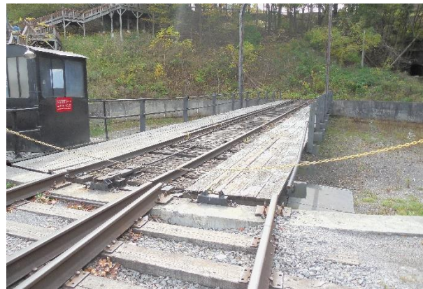
Pic 4: This 100' turntable at Frostburg is long enough for 1309, but approach tracks are too sharp until the track can be modified.
