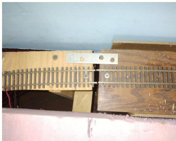
Photo 2: The adjustment screws and stopping plate. All are adjustable to align the track if needed
