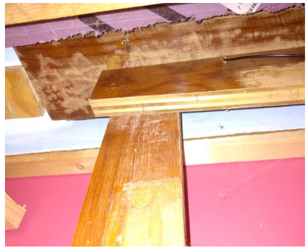
Photo 1: The elevator floor with stiffening spine, all 3/4" ply construction
