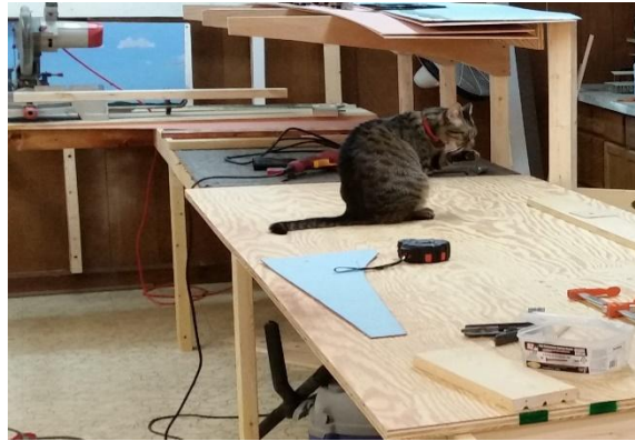
Figure 4 The inspector Luxor scrutinizing the progress.
