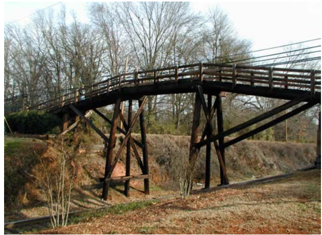
Oldest known wood RR footbridge—Waxhaw, NC
